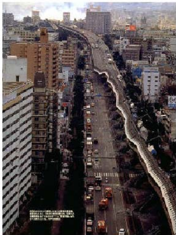
Figure 2.8 Collapsed Section of Hanshin Expressway
