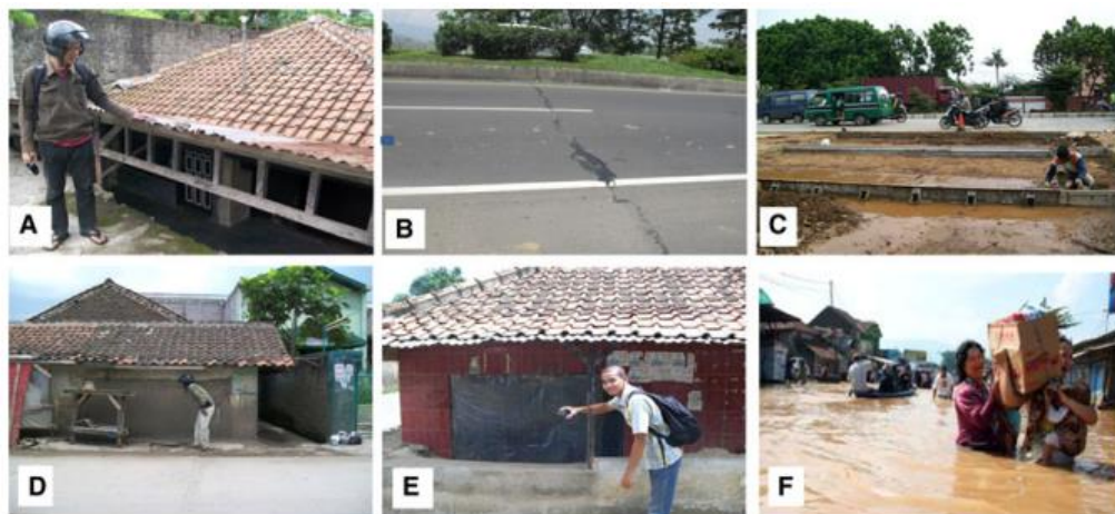
Gambar II. 2 Contoh Dampak Kerusakan Land Subsidence (II) (Abidin et al., 2013)
