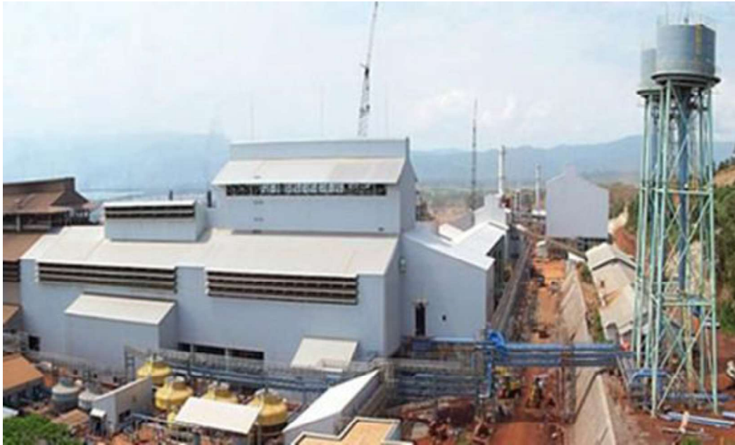
Figure 1.4 ANTAM's FeNi III Smelter Plant at Pomalaa, Southeast Sulawesi
