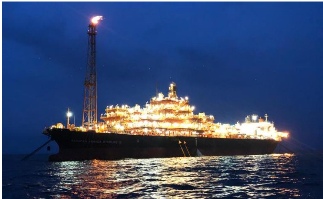
Figure I.9 FPSO KAS III at BD Field (Source: Company internal data)
