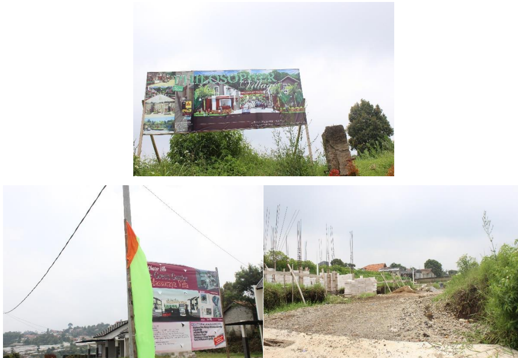
Gambar IV.7 Pembangunan Klaster Perumahan The Green Massuraya Village dan The Philosopher Village (Dokumentasi Pribadi, 2016)
