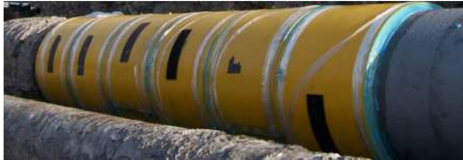
Gambar 2.33 Ilustrasi clock spring
