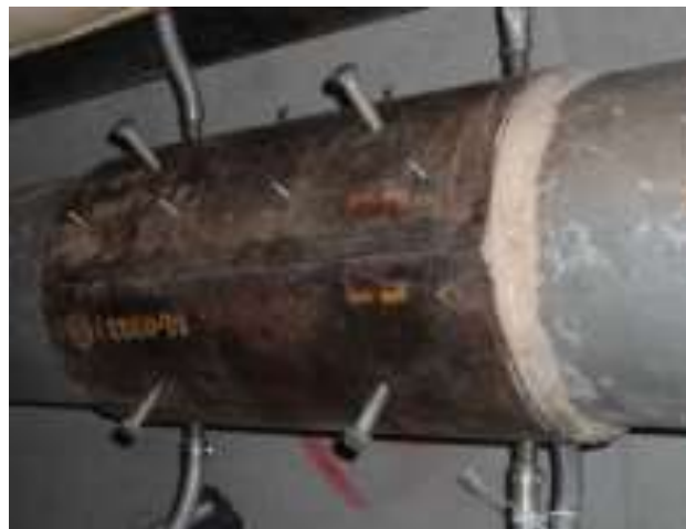
Gambar 2.32 Ilustrasi epoxy composition filled sleeve
