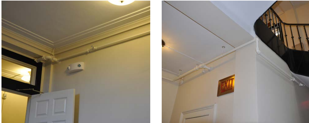
Gambar II.11 Sprinkler di Eno Memorial Hall, Connecticut Sumber: www.alfirect.com , diunduh 11 November 2014
